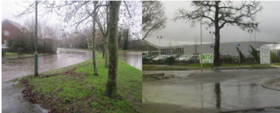
IMG013 Zebon Copse Balancing Pond overflows to roads Church Crookham
