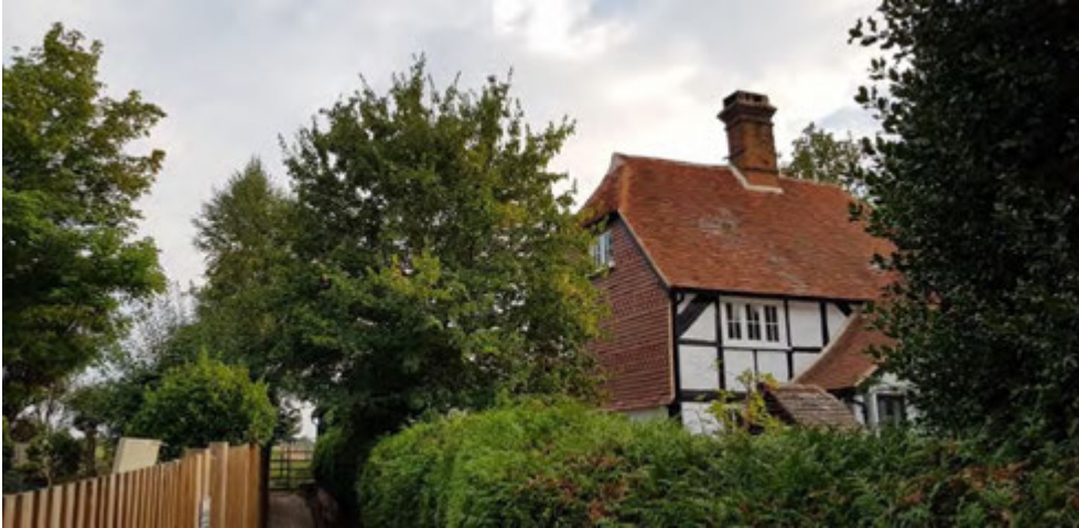
Figure 45 - Footpath 1 alongside Forge Cottage
