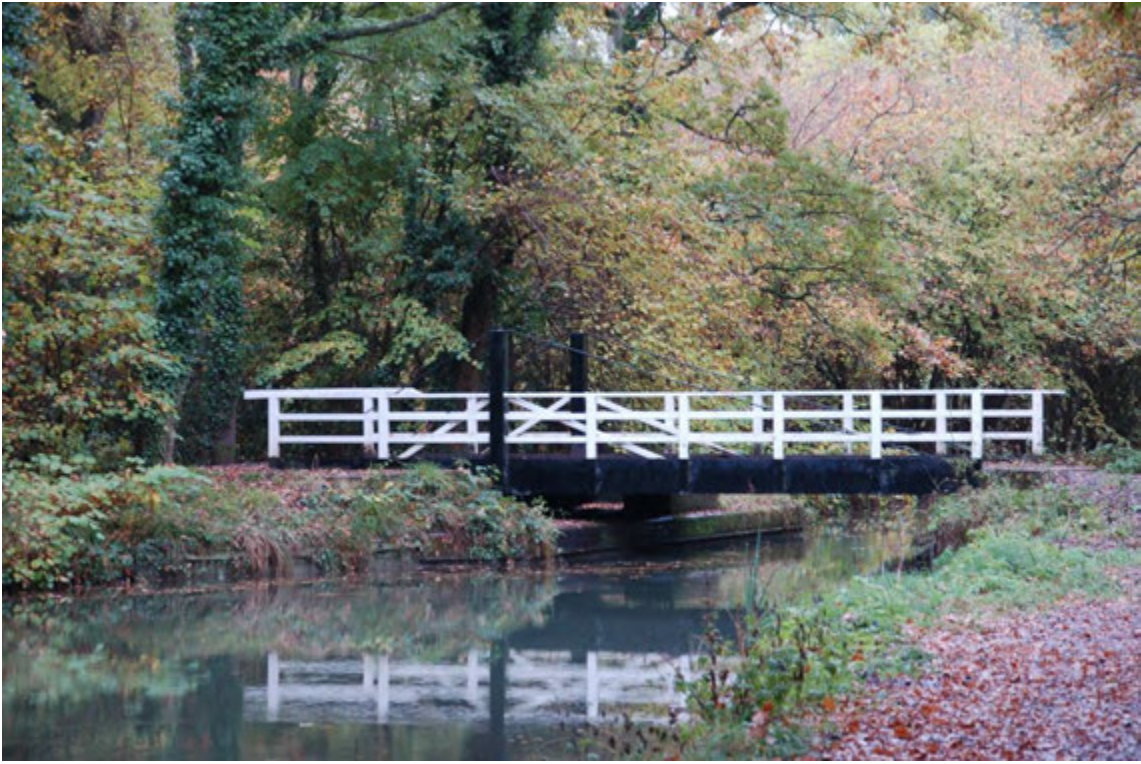
Figure 15 - The Swing Bridge
