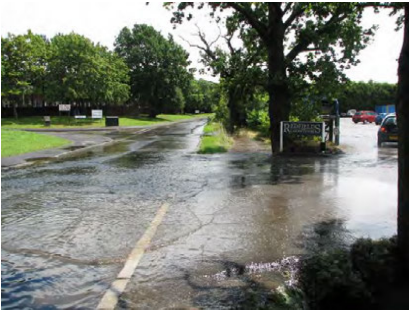
Figure 20 - The ditch across the entrance to Redfields Garden centre, July 2007
