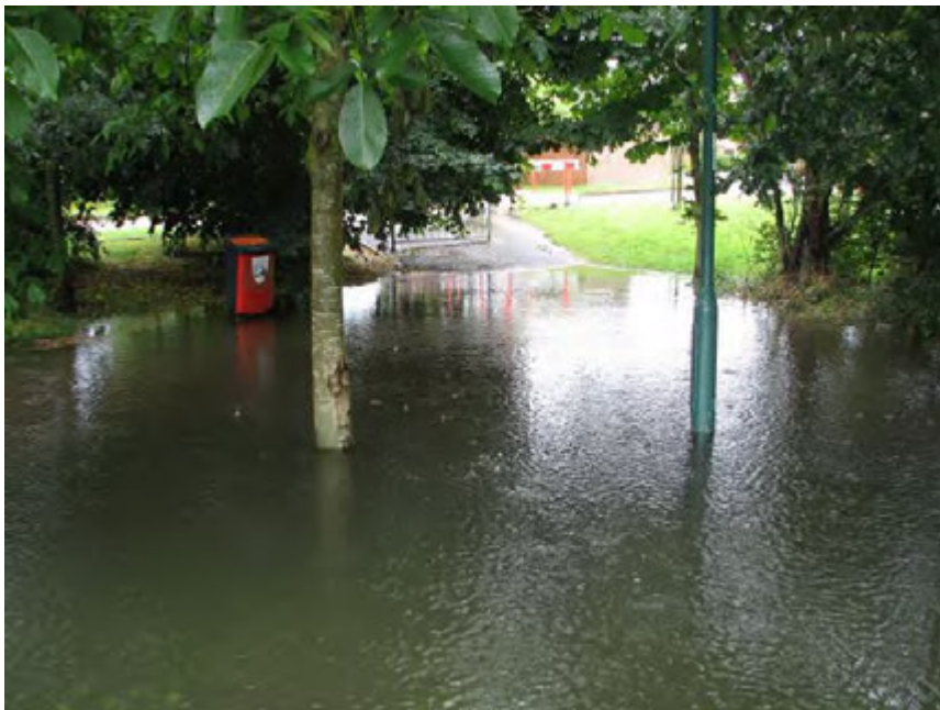
Figure 16 - Brandon Road balancing pond breach, July 2007 - Natural contours retained the water at the northern western edge of the pond area.
