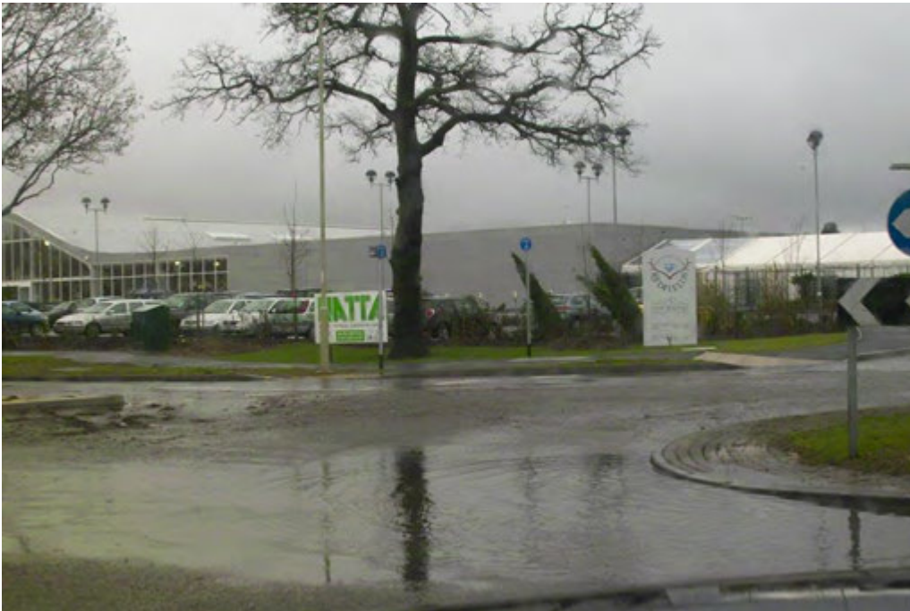
Figure 28 – The roundabout in front of Redfields Garden Centre
