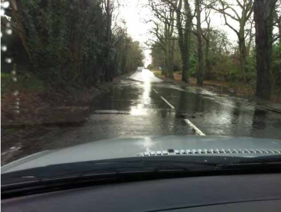
Figure 27 – Redfields Lane, approaching St. Nicholas' School and A287
