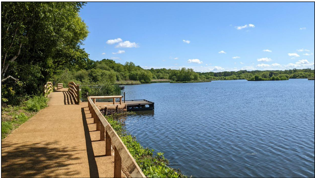
Image 1: The widened and resurfaced path at Fleet Pond
