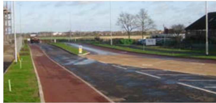
Stepped segregated cycle track
