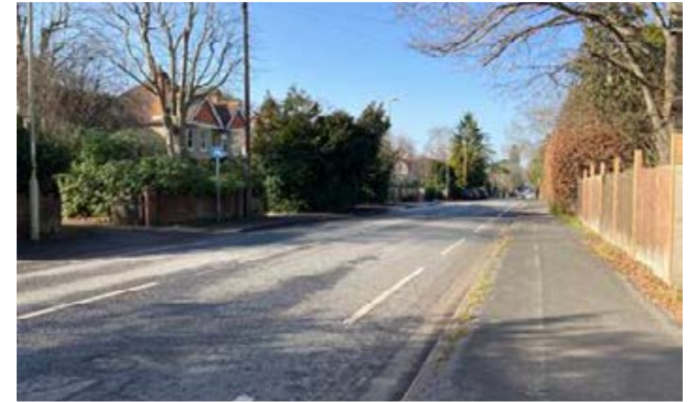
Narrow existing cycling facilities along Kings Road
