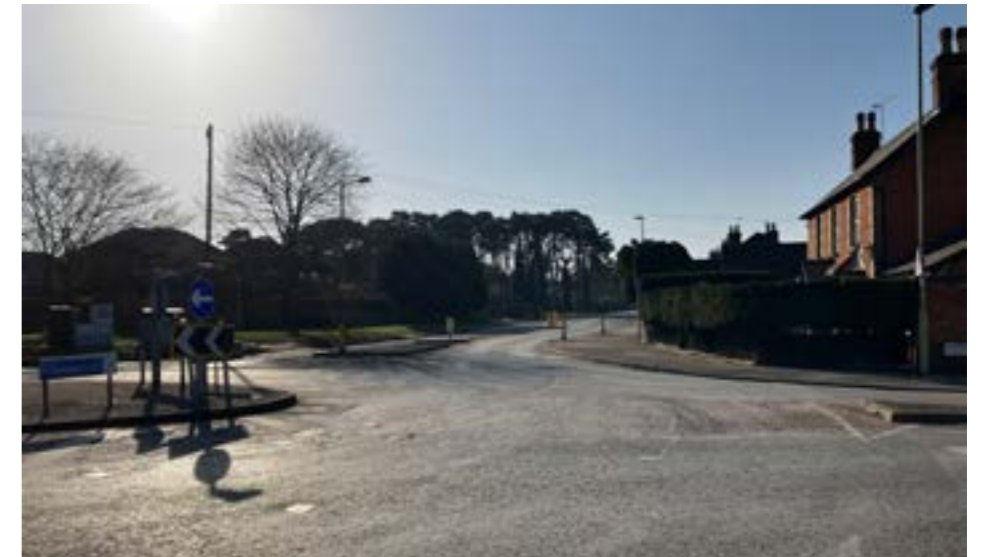
Opportunity to re-allocate extra carriageway space at Aldershot Road / Reading Road South roundabout
