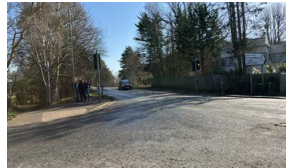
Extra carriageway space at the Aldershot Road / Kings Road junction
