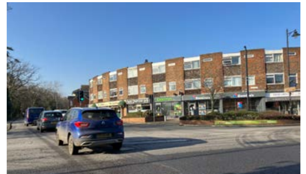
Opportunity to re-allocate extra carriageway space at Fleet Road / Crookham Road junction
