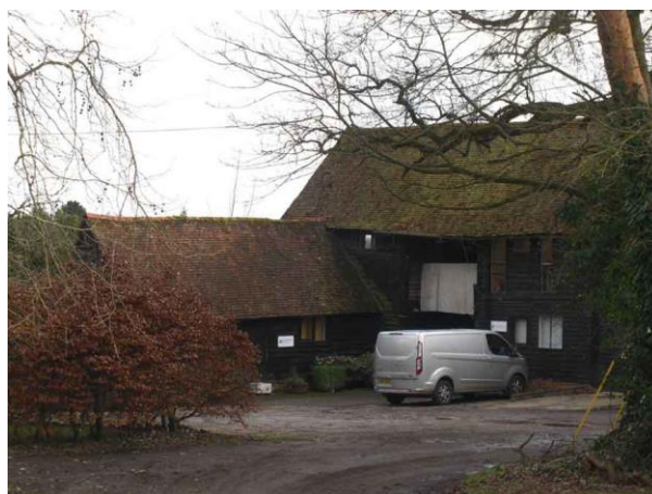
Conversion of traditional agricultural building for commercial use
