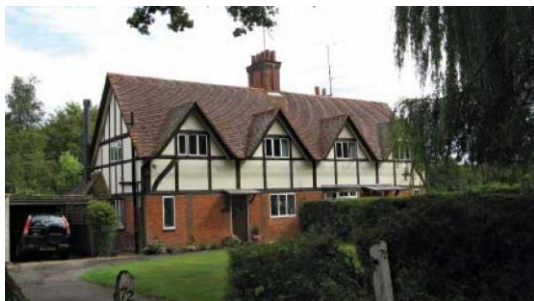
Cottages, Ridge Lane
