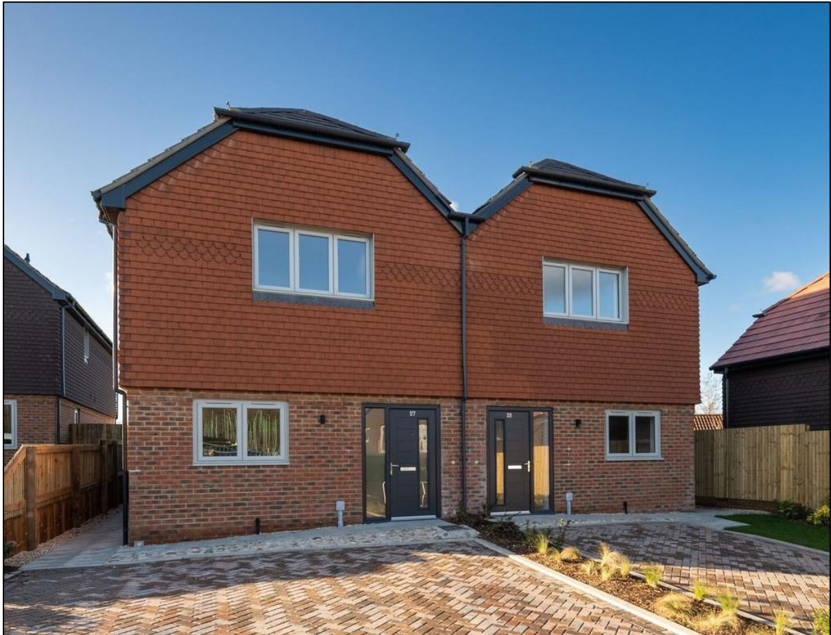
Image 7: Two-bedroom affordable homes delivered at Broden Stables, Crondall
