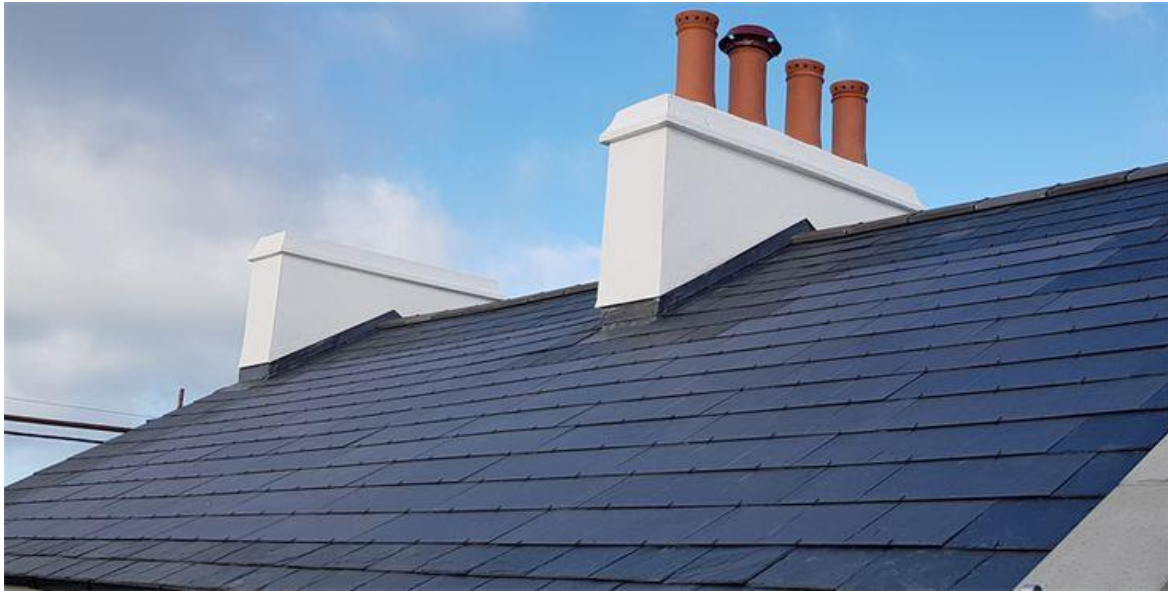
Image 4: Solar PV slates (Image credit: Wessex EcoEnergy)
